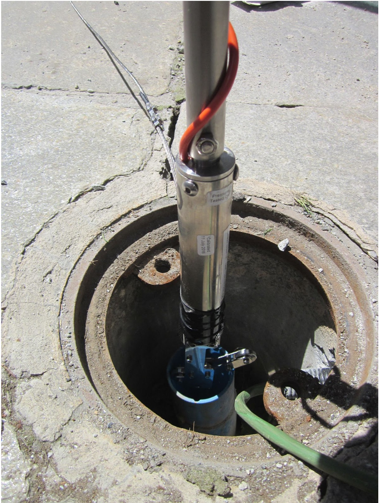
Figure 46 above shows how the network cable is secured to a spacer bar as the network chain is lowered into the casing. The wheel assembly slides into the sensor alignment guide built into the casing.
