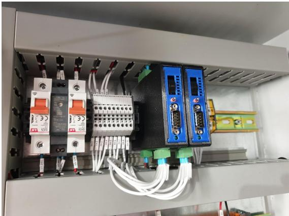
Figure-16 shows a DIN rail mounted VibWire-301 Installation.
